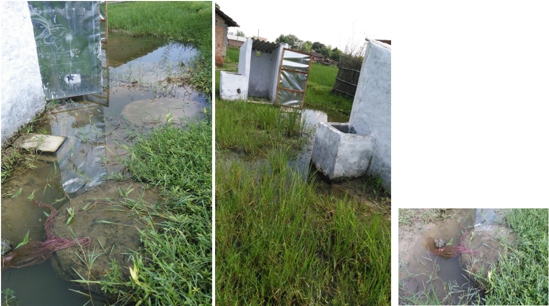
Sahib ganj District Bada Tufir Village Latrines constructed by PHED
